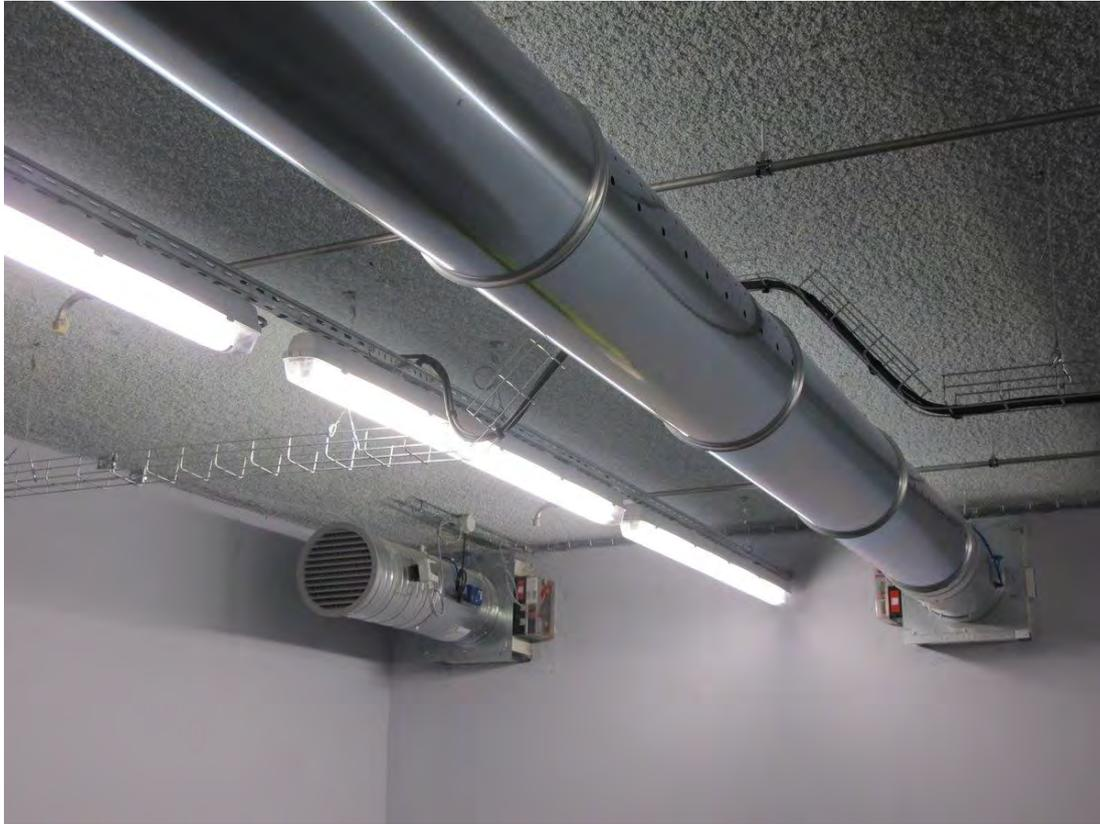
This special air distribution process is sometimes used in the automobile and aeronautical industries when a high level of homogeneity in climatic conditions is desired for large volumes. The air supply duct has perforations calculated to obtain very high induction, ensuring that the ambient air moves with a lower blown airflow rate.
